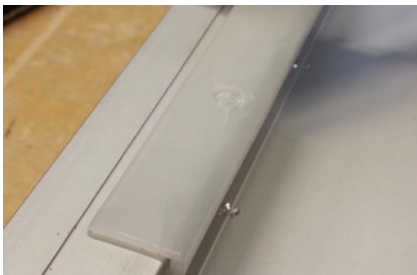
Fitted profile secured by plastic screw, head removed.
