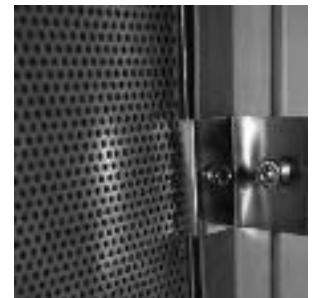
panel fixed with bolt lock
